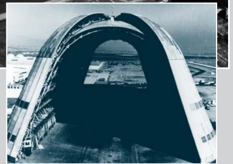
A view of the huge dirigible hangar with doors open at both ends. The hangar was erected in 1931–33 and covers eight acres.
