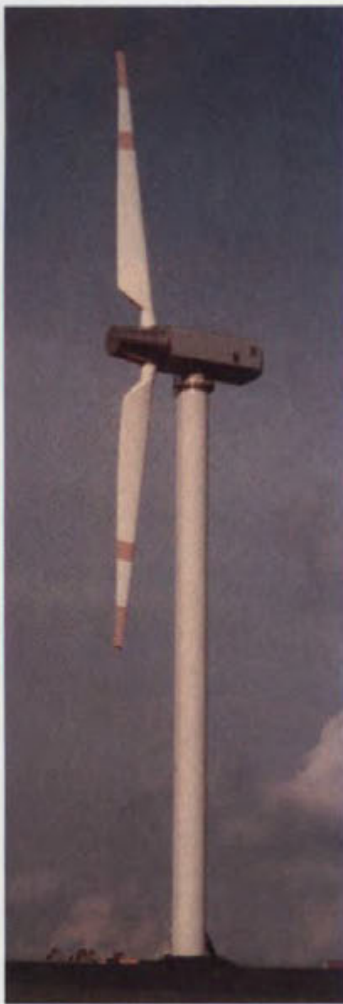
Figure 4. 4MW WTS-4 Wind Turbine (257 ft. diameter).
