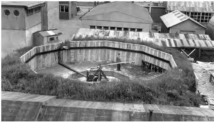
Drees, Gerard Verhage and Will Kupers developed the ramjet-powered Kolibrie, with support from the Centre, including testing the rotor system at NLL Amsterdam. (NLR photo)
